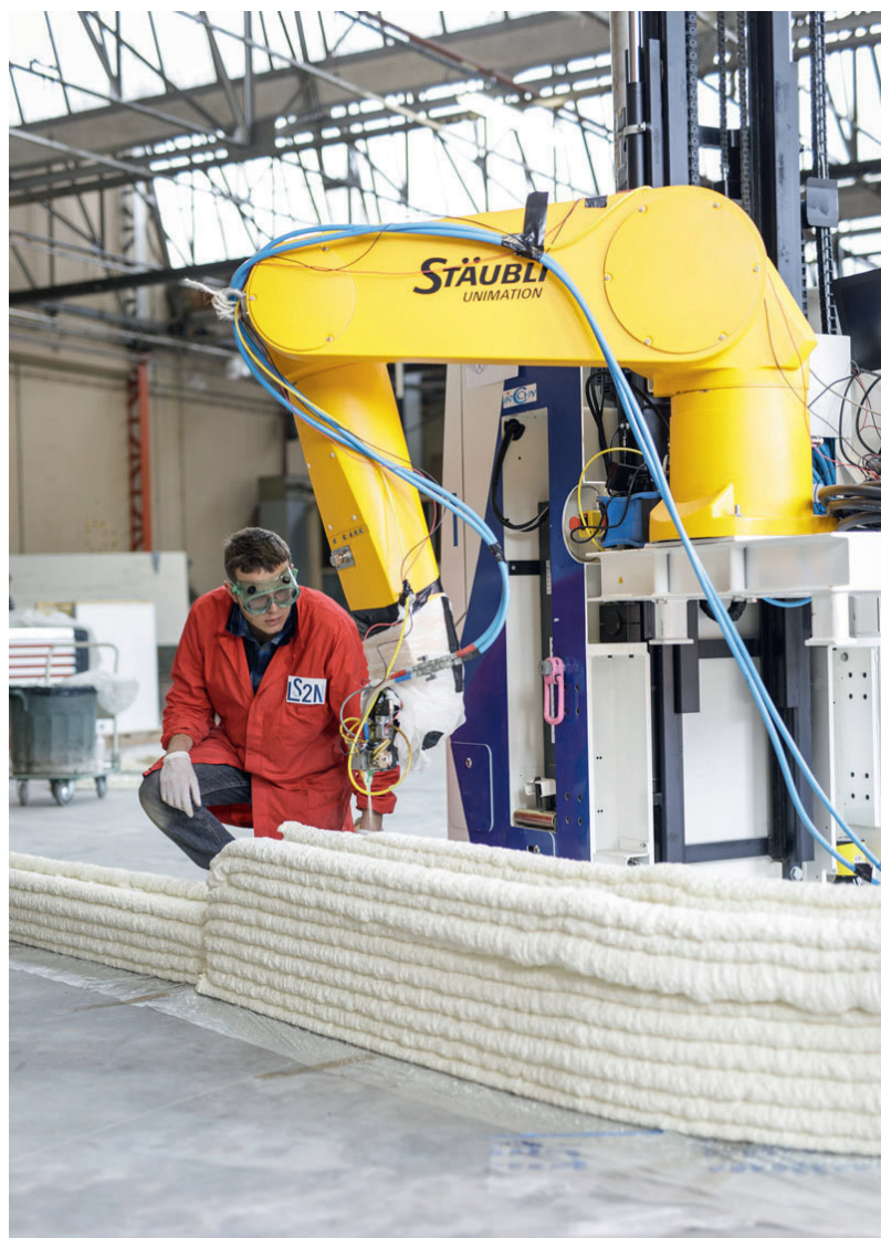
The Batiprint 3D robot performing structural work for a 95 m 2 building.
